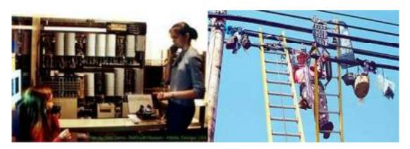
Voice call 1984. A touch tone phone with battery in the central office on a mechanical switch would push 7 digits for the number of the person you wanted to call. The central office sends ring current to ring bells in the touch tone phone. When answered, the central office provides DC current to both parties. When one of them spoke, current is sent to the phone on the other end. The ear piece converts the current into analog voice where the ear could hear it.
