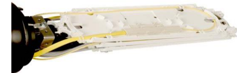
Splitter in splice tray
